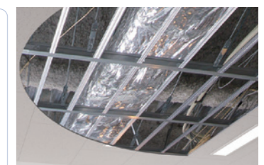
Our own anti-seismic ceiling construction technique
