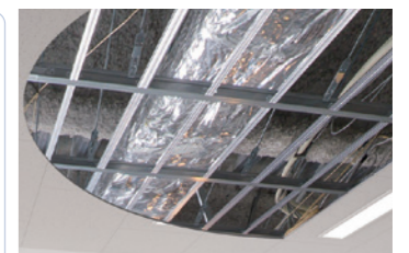
Our own anti-seismic ceiling construction technique
