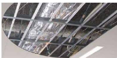
Our own anti-seismic ceiling construction technique
