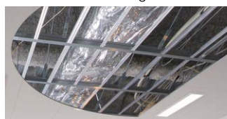
Our own anti-seismic ceiling construction technique
