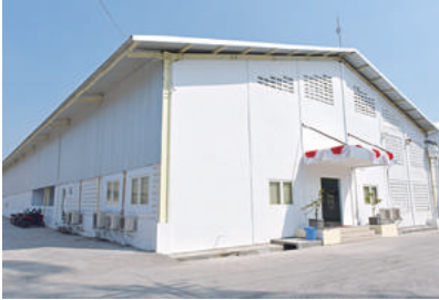
Appearance of the factory of PT. Daiken Dharma Indonesia
